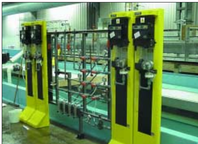
■ A pre-fabricated multiple-use-point NaOCl dosing system with panel-mounted ejectors and gauges.
