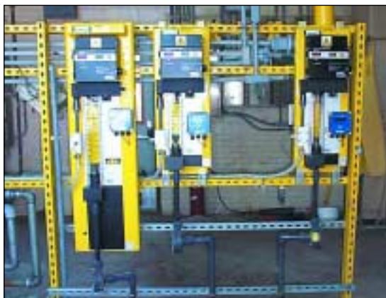
■ Three vacuum dosers of varying capacities, with alarms for high and low vacuum and flowmeters.
